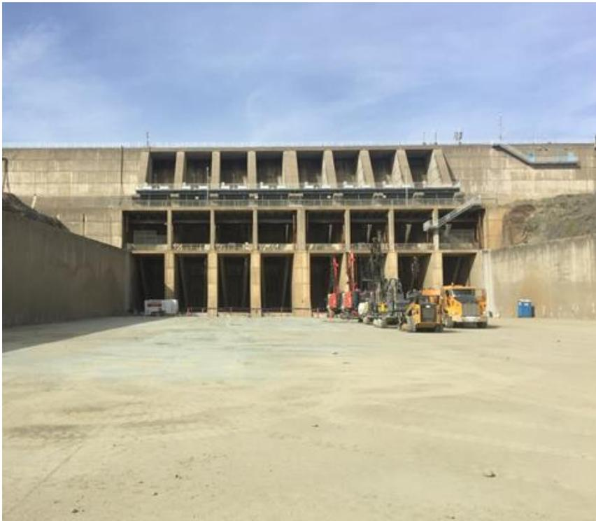
Figure 1. Main Spillway Slab and Gate Structure.
