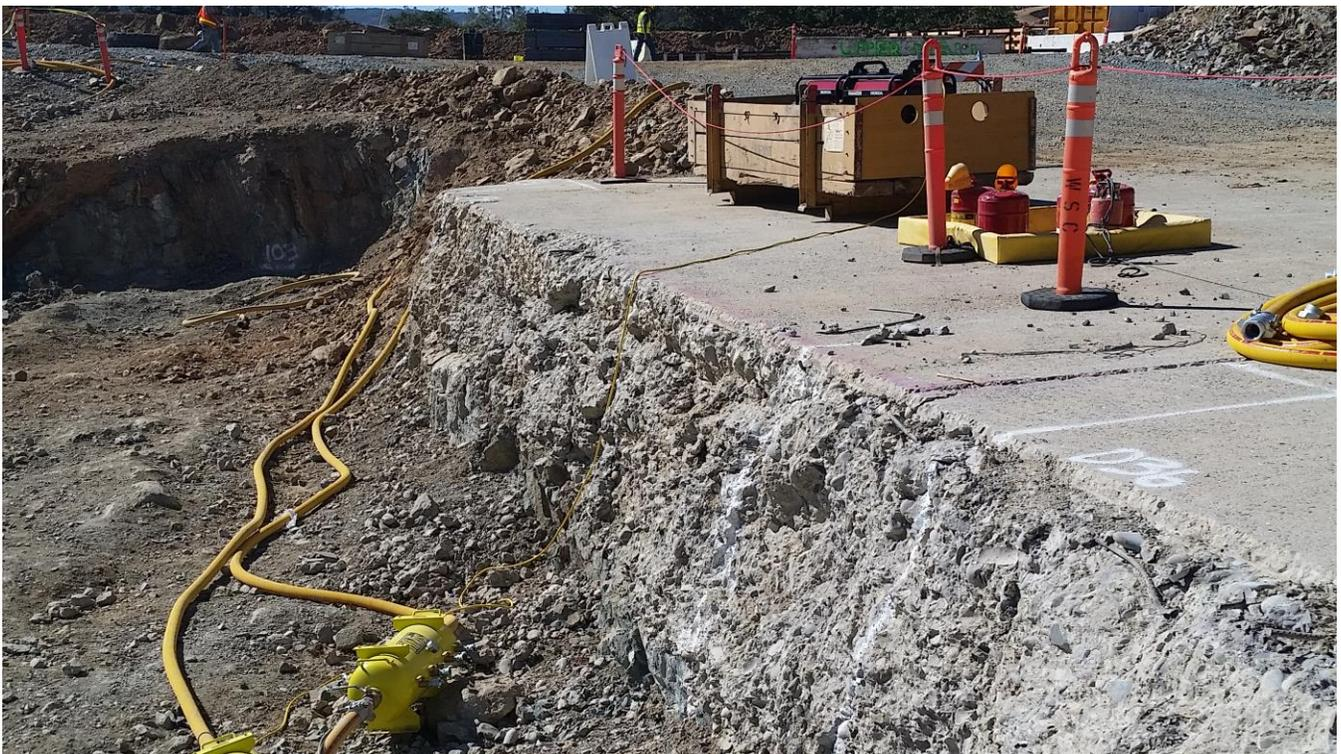
Figure 9. Exposed expansion/contraction joint 18-inches from the nearest blast holes.
